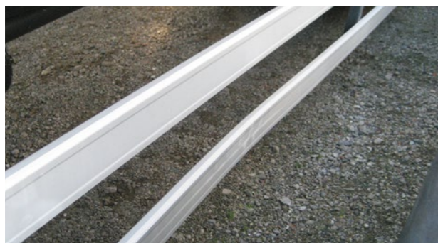
🔧 Bike racks: Deformation within economic repair
