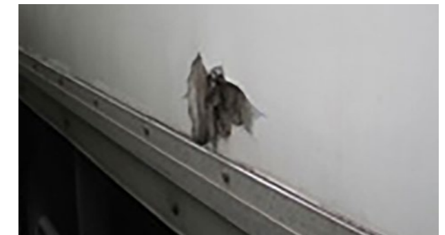
Wood side panels: Damaged wood support \geq 20 cm
