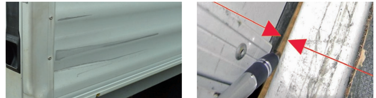
Deformations in the rails not beyond economic repair, closure not possible or not sand-proof
