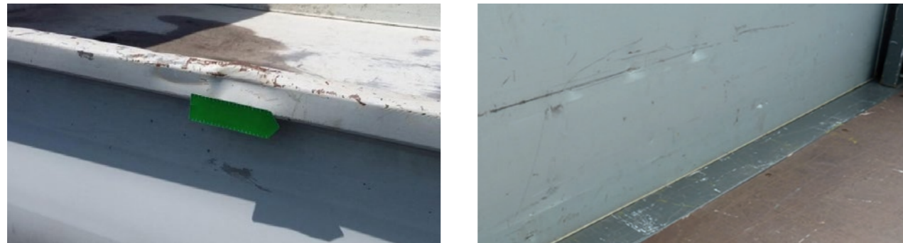
Faint scratches, rail deformations with a repair time \leq 1 h
